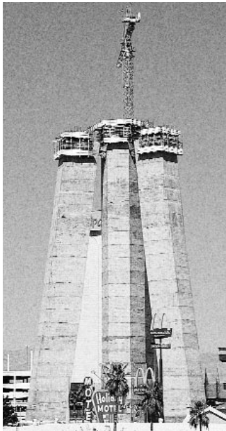
The Grand Casino tower in Las Vegas used Power Team hydraulics to counteract deflection and control twist in the tower fabrication. They used six Power Team C1506CL 150 ton locking collar cylinders powered by Power Team PE553 pumps.
