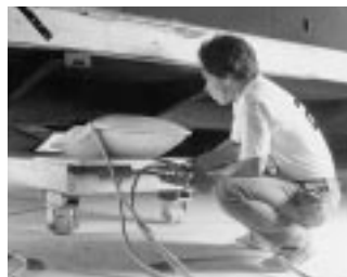
Power Team inflatable jacks raise a 33,000 lb. modular home section, providing clearance for installation of temporary wheels for transport.
